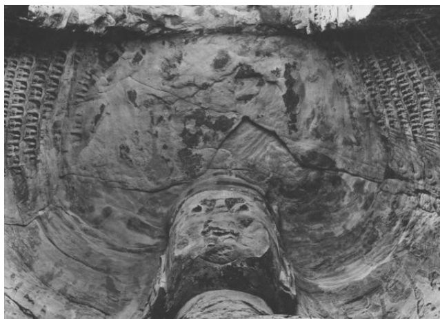
Figure 8 – Vault of Cave 17
