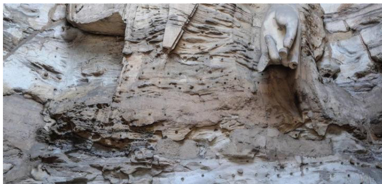
Figure 3 – Severe weathering of mudstone
