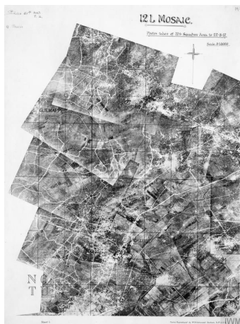
Figura 4: Mosaic of aerial photographs of the trenches taken during the First World War
